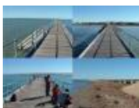
Various shots of the Port Germein jetty.
