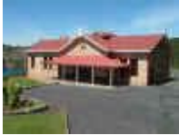
The water Pump House at the Blue Lake.
